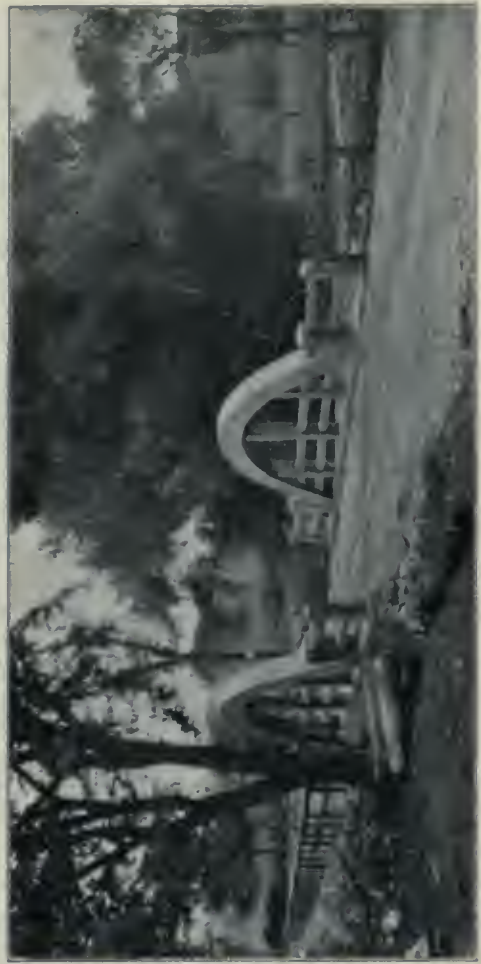
Concrete Arch with Suspended Floor in Halton County—Greater head room is possible by means of this form of construction.
